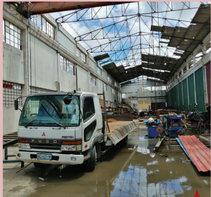
Macsteel Group suffered great damages
